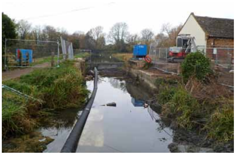
Work on replacement Ocean swing bridge (2011) © John Grayson, Geograph (CCL)
