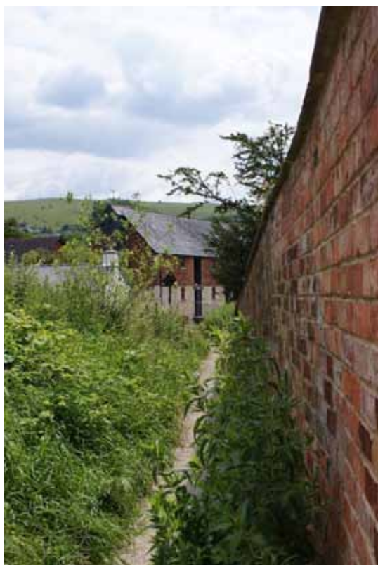
Route of the railway line linking the canal with the mill © Sara Chardin
