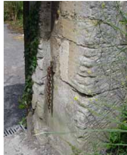
Grooves in the stone archway made by towing ropes © Jenny Lunn
