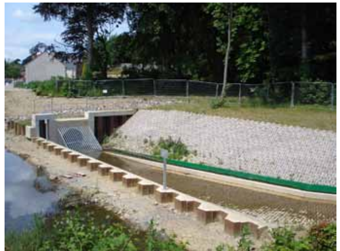
Hydro electric scheme installed at Dudbridge Lock © Jenny Lunn
