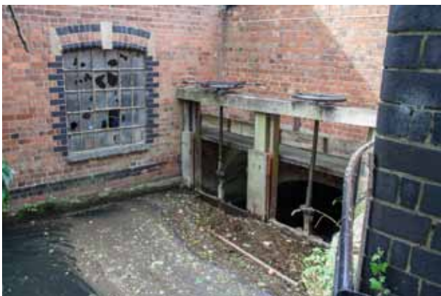
Sluices at Ryeford © Nick Bird
