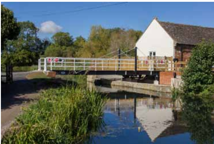
New Ocean swing bridge in place © Nick Bird
