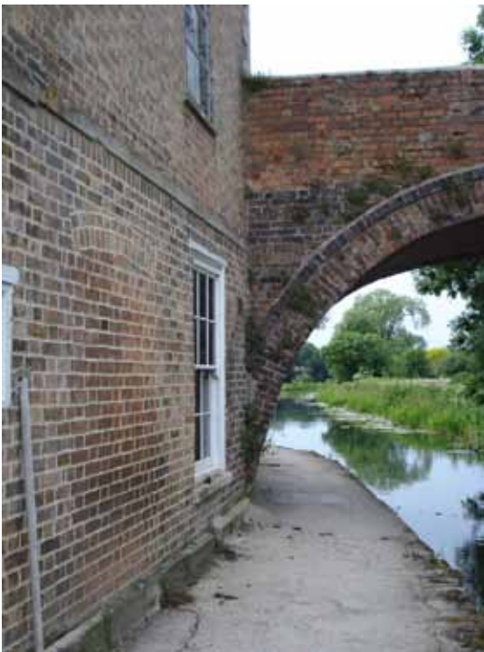
Old doorway in the brickwork of Nutshell House © Jenny Lunn
