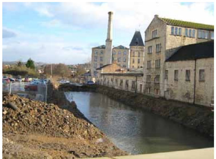
Ebley Mill in 2008 showing canal restoration in progress © David Stowell, Geograph (CCL)
